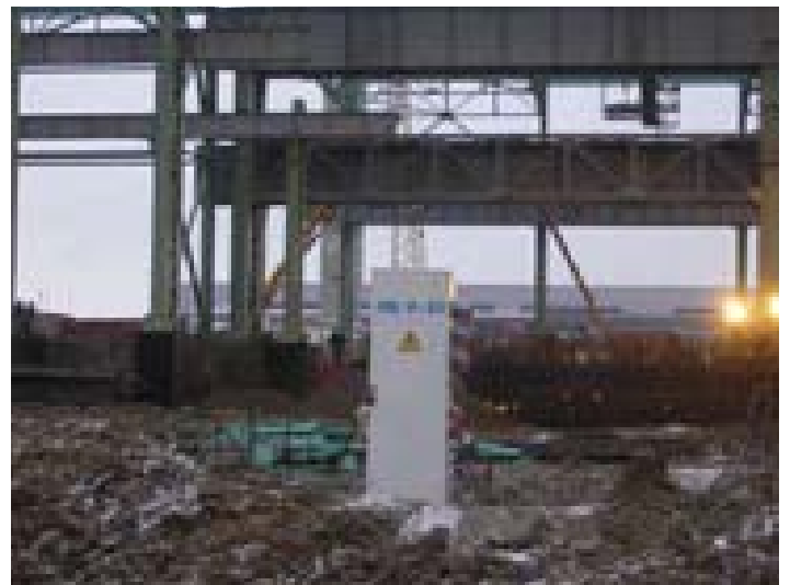
OKM (United Metallurgical Company), Vyksa – Russia
