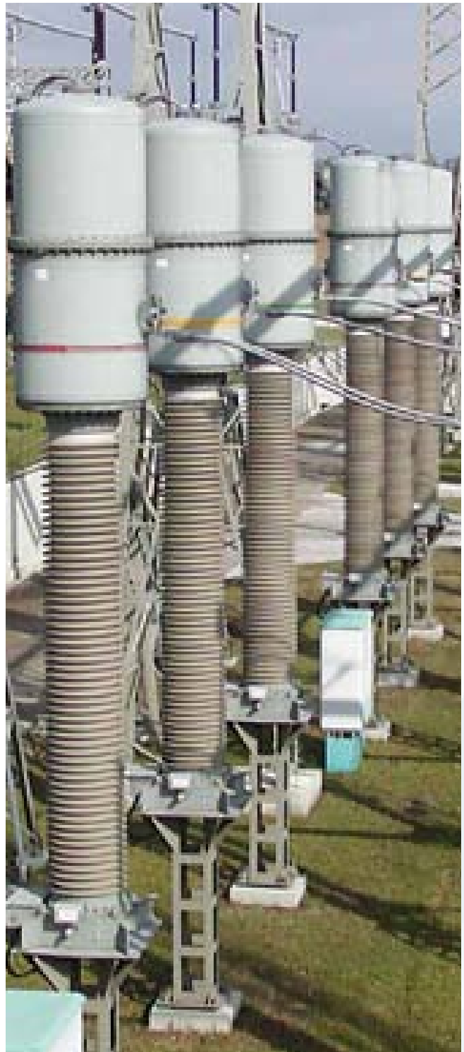
800kV, SF 6 insulated combined instrument transformer (extended accuracy range)
