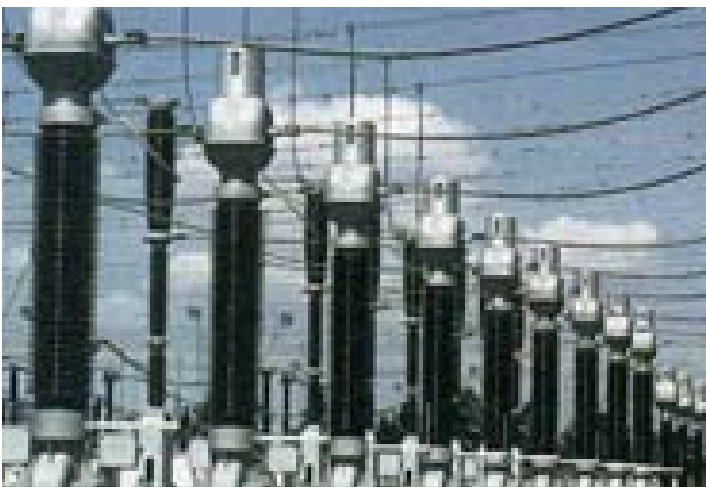
245kV, Oil insulated combined instrument transformers
