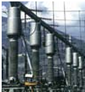
245kV, SF 6 insulated, combined instrument transformers
