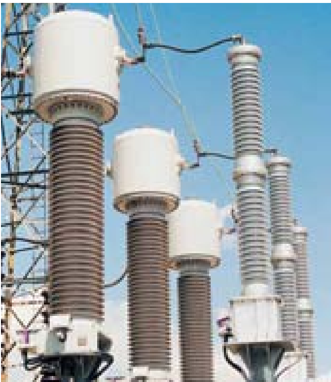
245kV, SF 6 insulated current transformers
