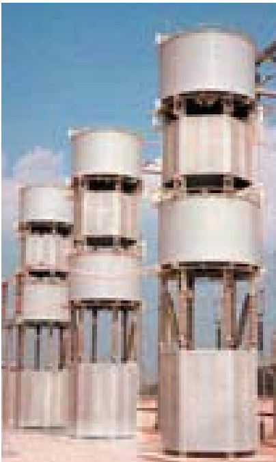
138kV, variable impedance series load flow reactors
