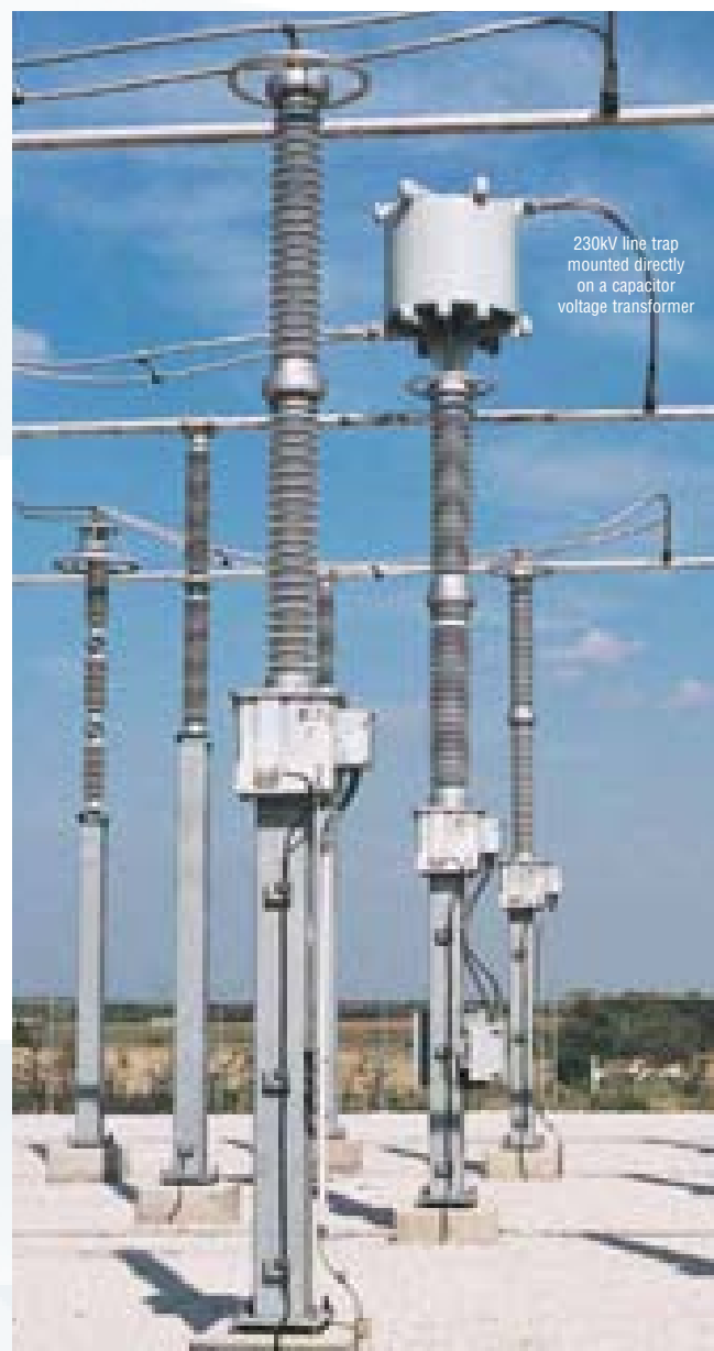
230kV oil insulated capacitor voltage transformers
